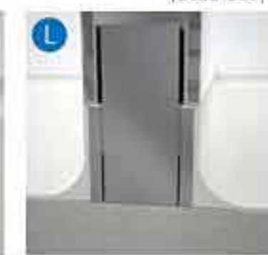
Floor at Framed Wall
